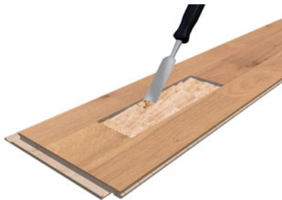
Chisel out the strip and 2 mm of the intermediate layer using a wood chisel.
