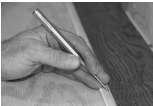
Fig. 6 Nail is completely lowered
