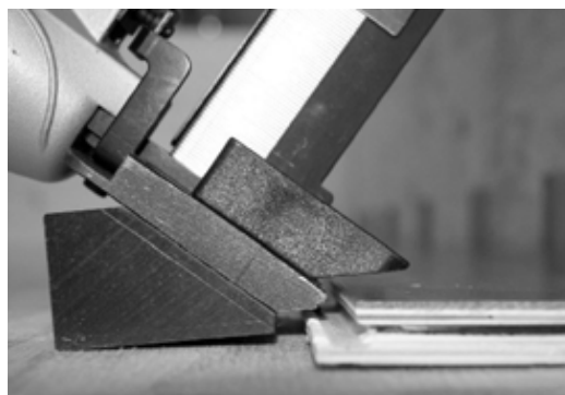
Fig. 9 Nail gun lifted over the locking element
